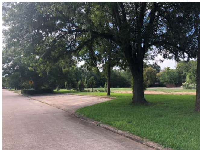
Current site condition with structure demolished
