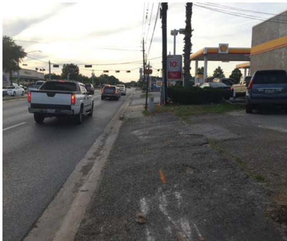
Existing FM 2351 Intersection
