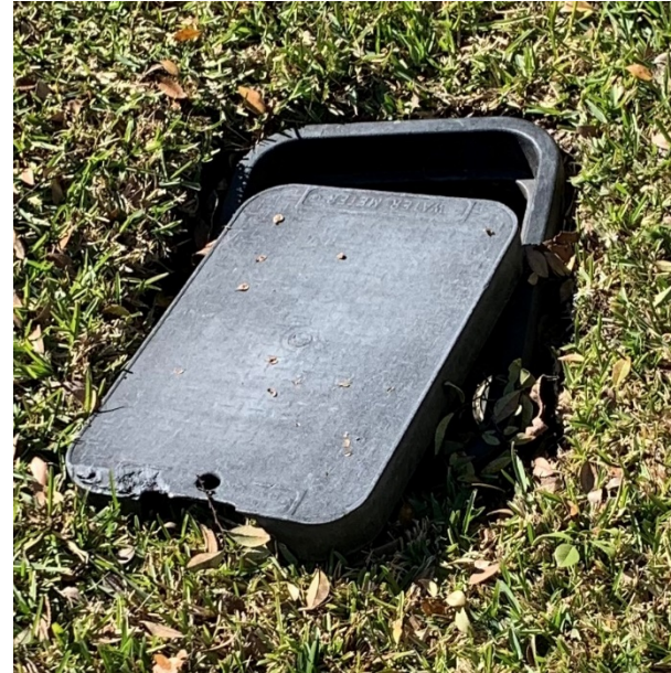
Broken Box and Box with Concrete Lids
