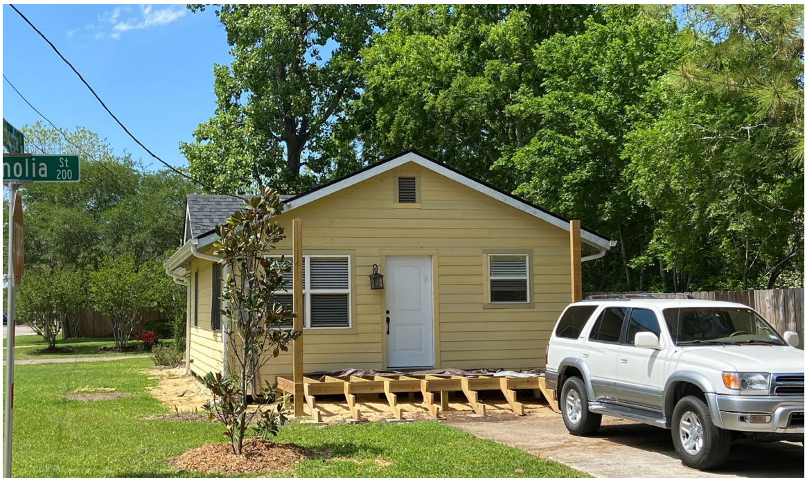
Code Enforcement Photograph of new construction
