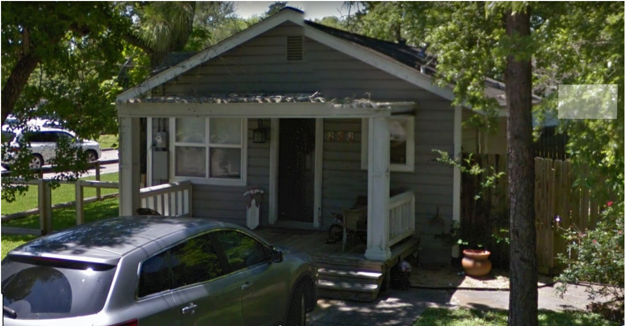
Google Street View Picture of Nonconforming structure - "Grandfathered"
