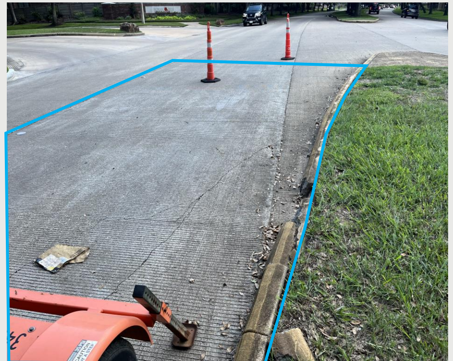
Area #1 - 7" Concrete RR - 4,480 SF
