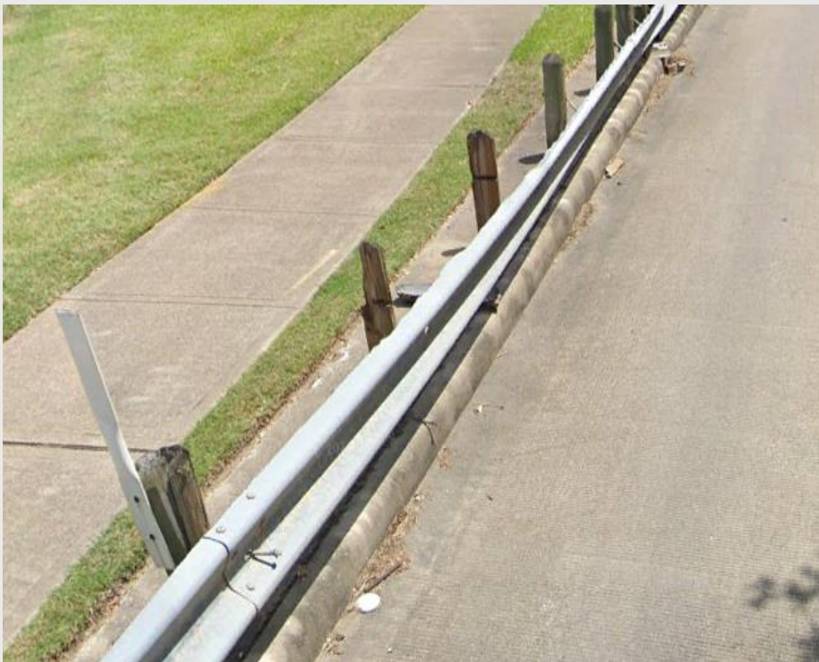
Area #4 - Guardrail Replacement - 120 LF
