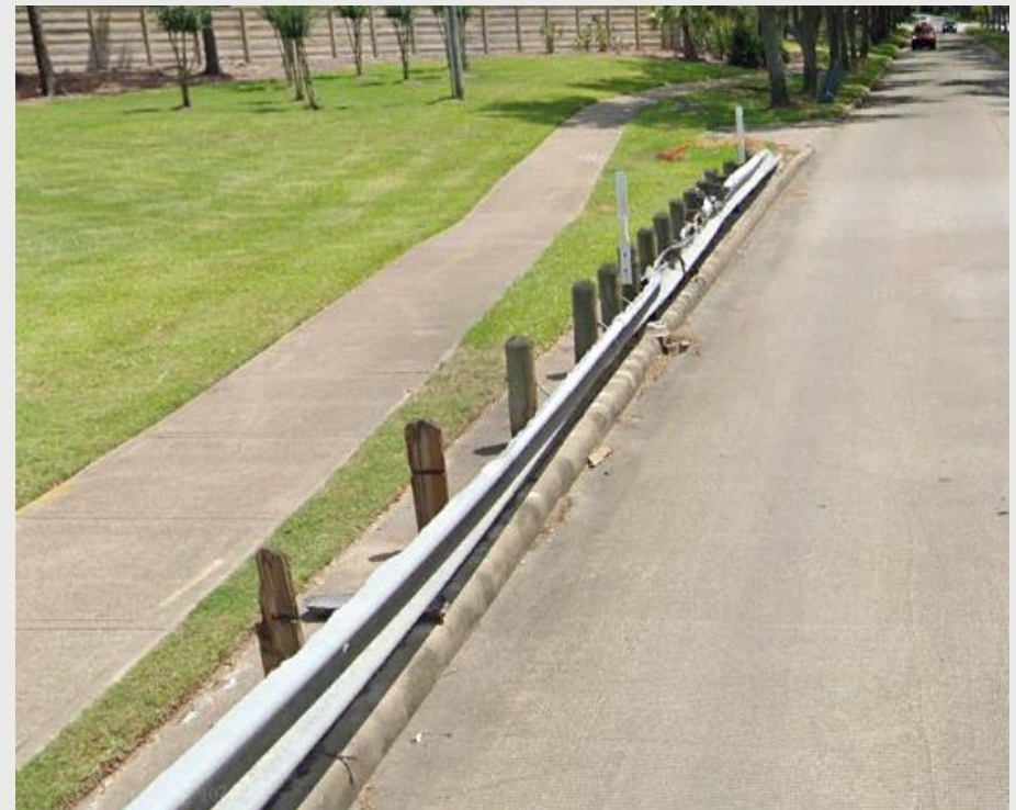
Area #4 - Guardrail Replacement - 120 LF
