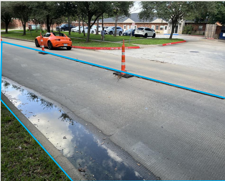
Area #1 - 7" Concrete RR - 4,480 SF
