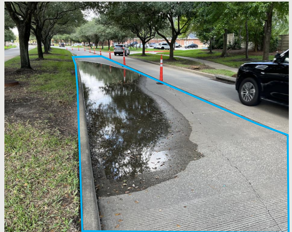
Area #1 - 7" Concrete RR - 4,480 SF
