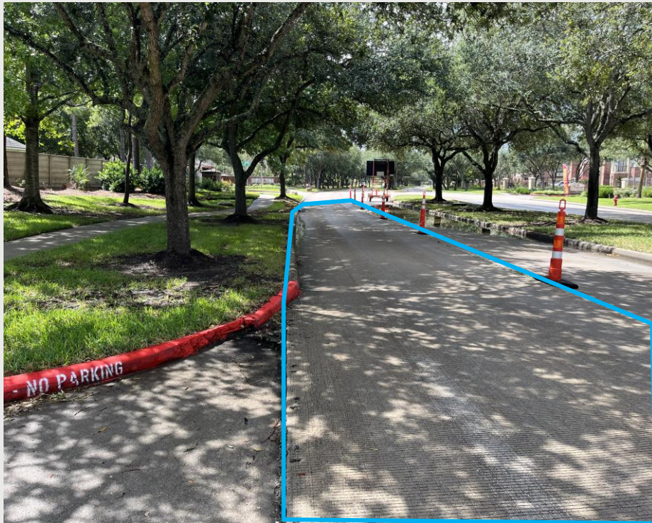
Area #2 - 7" Concrete RR - 4,354 SF
