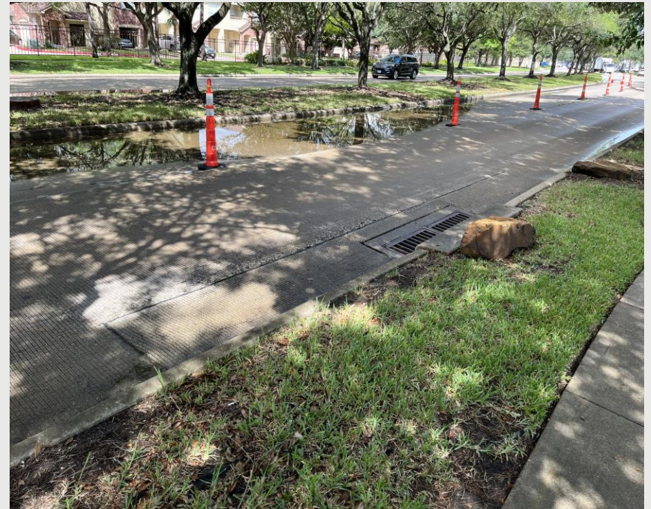
Area #2 - 7" Concrete RR - 4,354 SF
