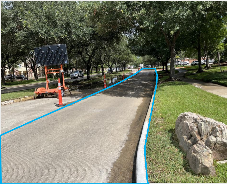
Area #2 - 7" Concrete RR - 4,354 SF
