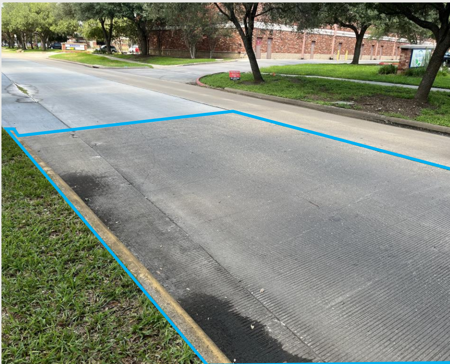
Area #1 - 7" Concrete RR - 4,480 SF
