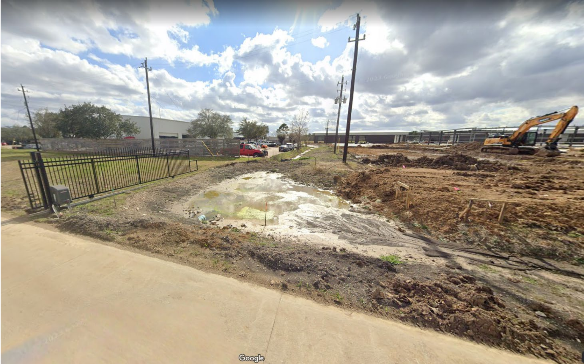
View from Industry Park Entrance...back of Eagle Transmission and future location of Buildings 3 and 5
