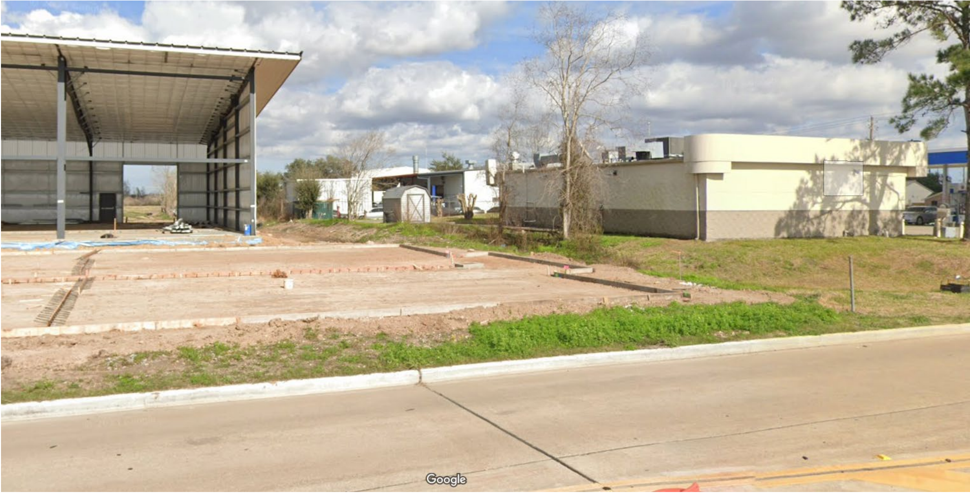
View from Timber Creek Drive Entrance...back of Chevron and edge of Building A
