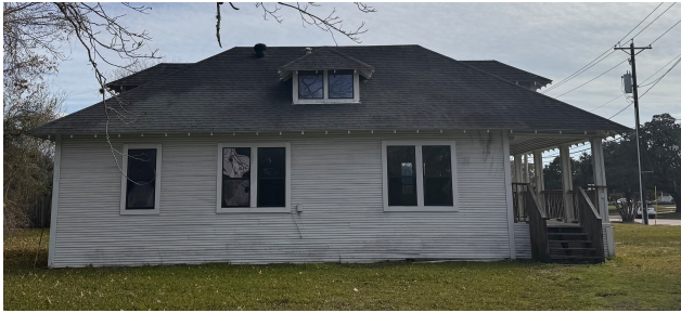
SIDE FACING NW AND CASTLEWOOD
