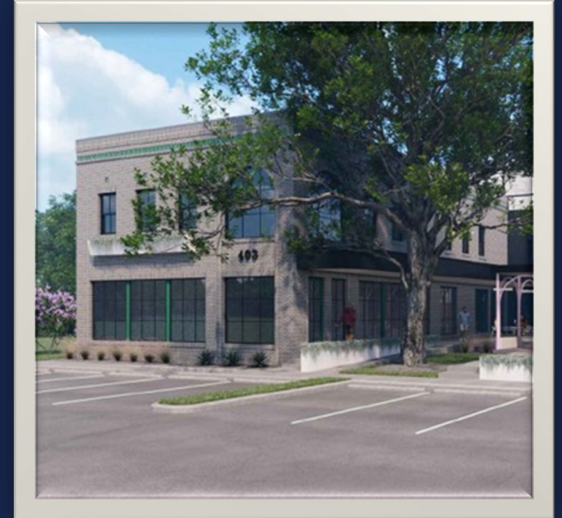
Augusta Kelly Office Building 403 Laurel
