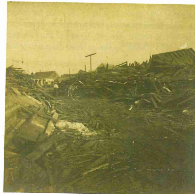
L & 15 th St. showing cut through the debris under which thousands of bodies were found. Photo by E. D. Aiken, 1900. Courtesy of Rosenberg Library, Galveston, Texas.
